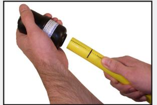
**8** Stab pipe completely into fitting so that the mark on the pipe is within 1/8" from the fitting entrance.
